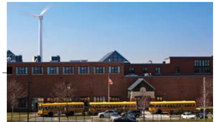
The City of Medford, Massachusetts owns a Northern Power Systems Northwind 100 wind turbine sited at McGlynn Elementary & Middle School. PIX16730/Northern Power Systems.
